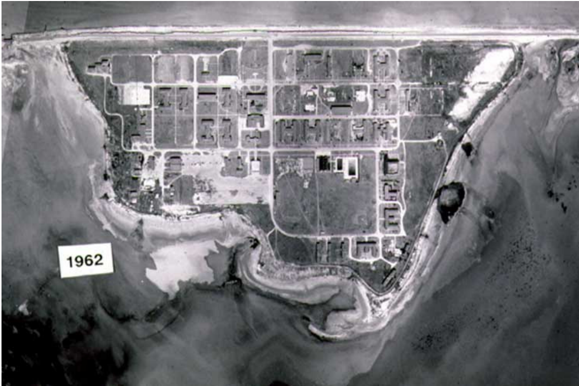
Illustration No.2.3 WARD ISLAND AFTER PARTIAL DEMOLITION OF WORLD WAR II BUILDINGS
