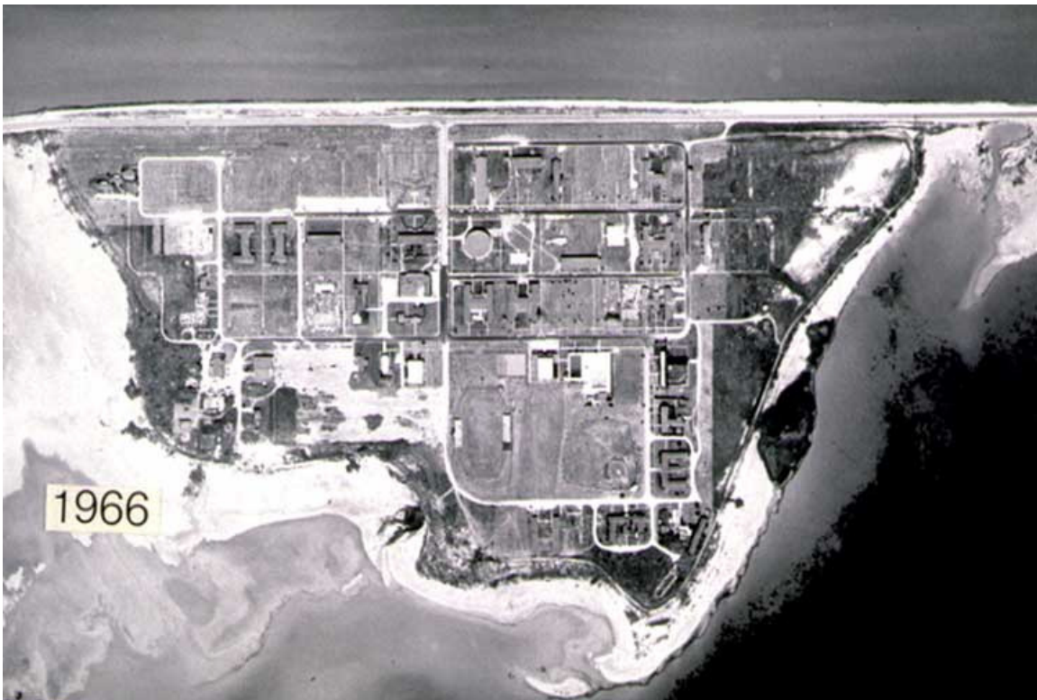
Illustration No. 2.4 START OF NEW CONSTRUCTION FOR THE UNIVERSITY
